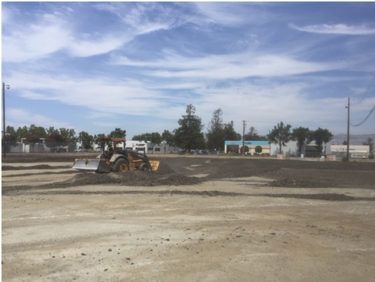
Parking lot – spreading fill
